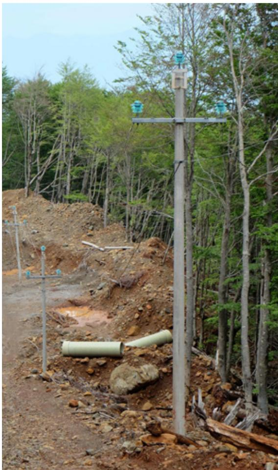
Figure 17: Erosion around the penstock
