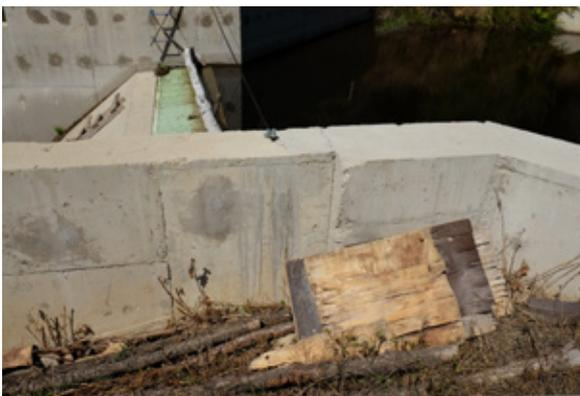
Figure 22: An appliance potentially used for blocking the fish pass on Stanisar intake
