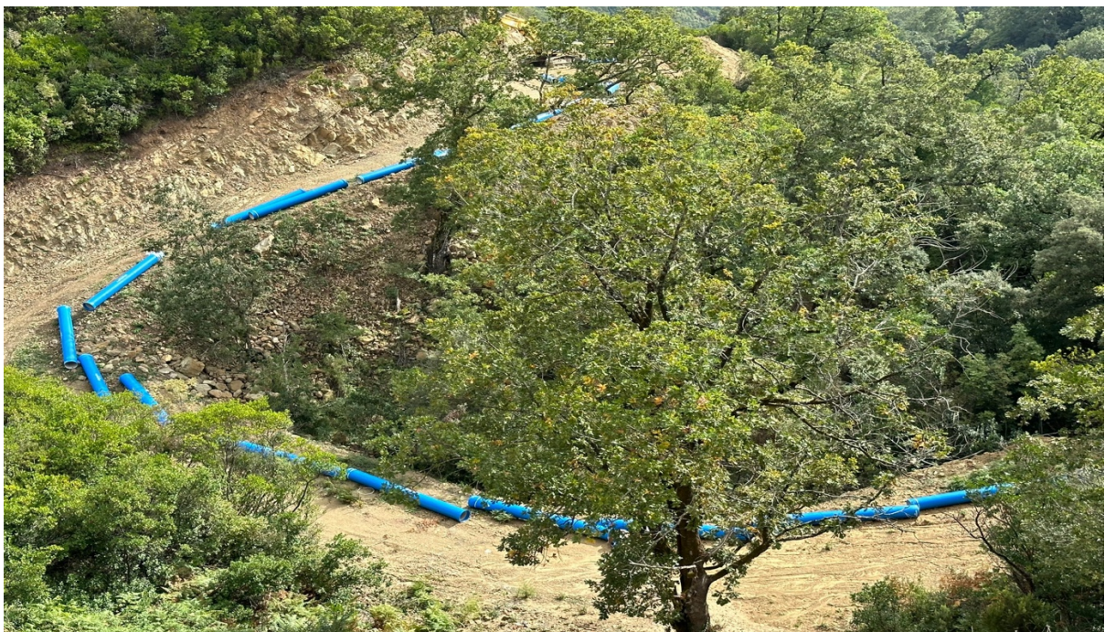
Figure 6: The distribution of the pipes along the pipeline route © U. Eichelmann
