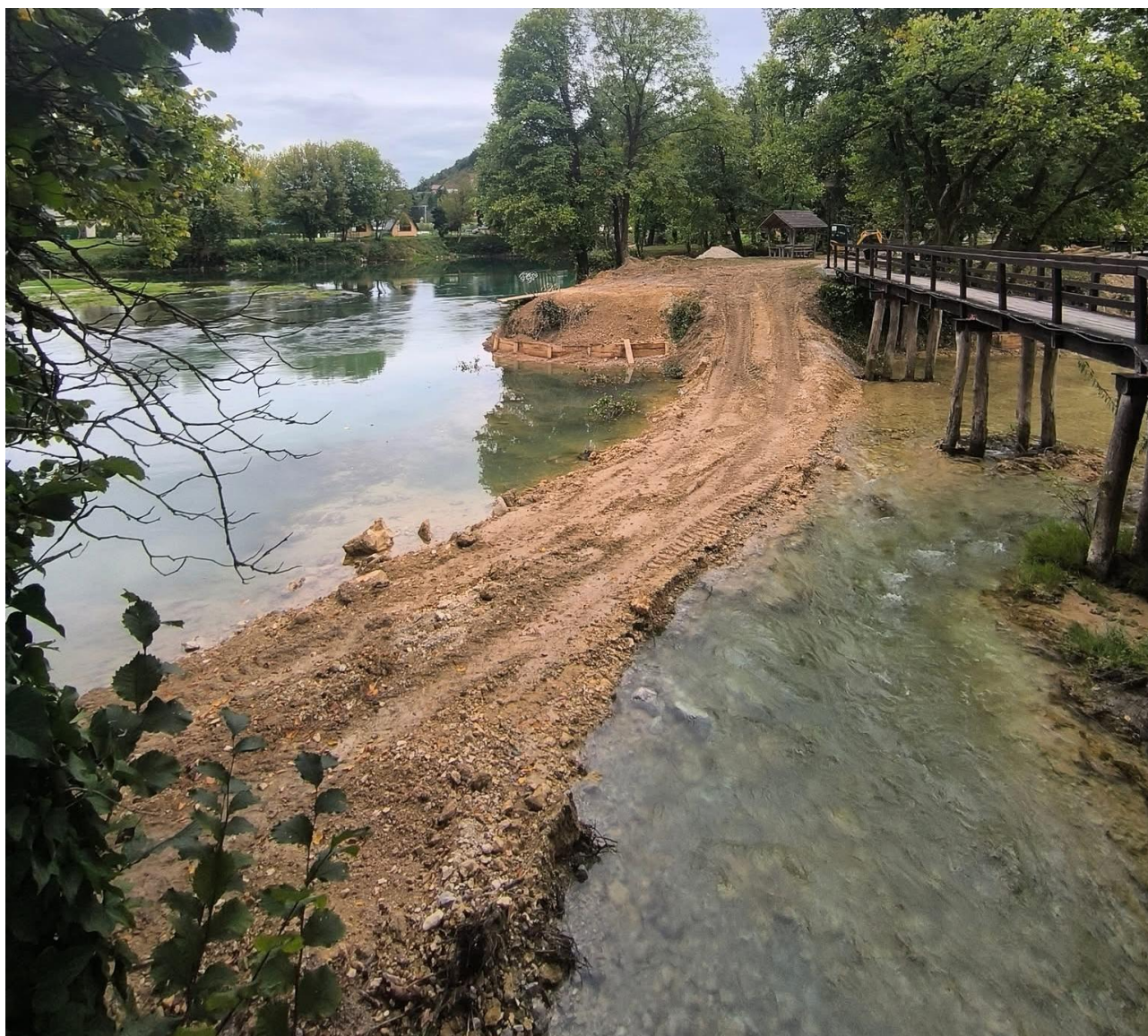
Figure 25: Newly built crossing (picture: Anes Halkic)
